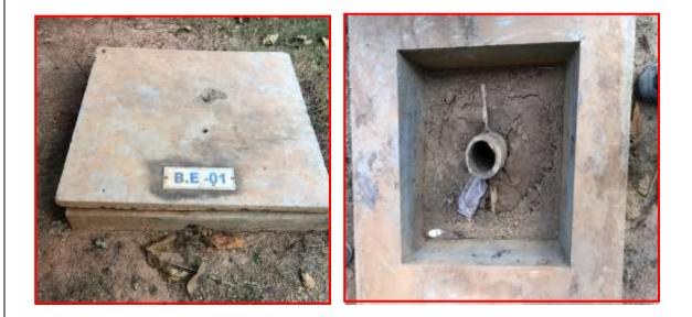
It is observed that body earth is conventional type. University's Earthing system must be in better condition as it is prone to malfunction and gives rise to harmonic and multiply the same into the electrical network.
